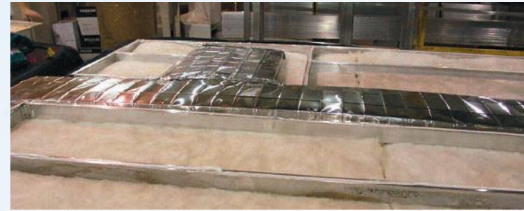
2" x 3" Aluminum floor studs
