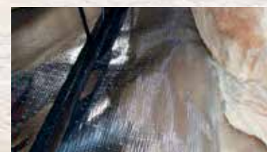
R-38 Radiant shield Thermo-foil wrap through ceilings, underbellies and under front caps.
